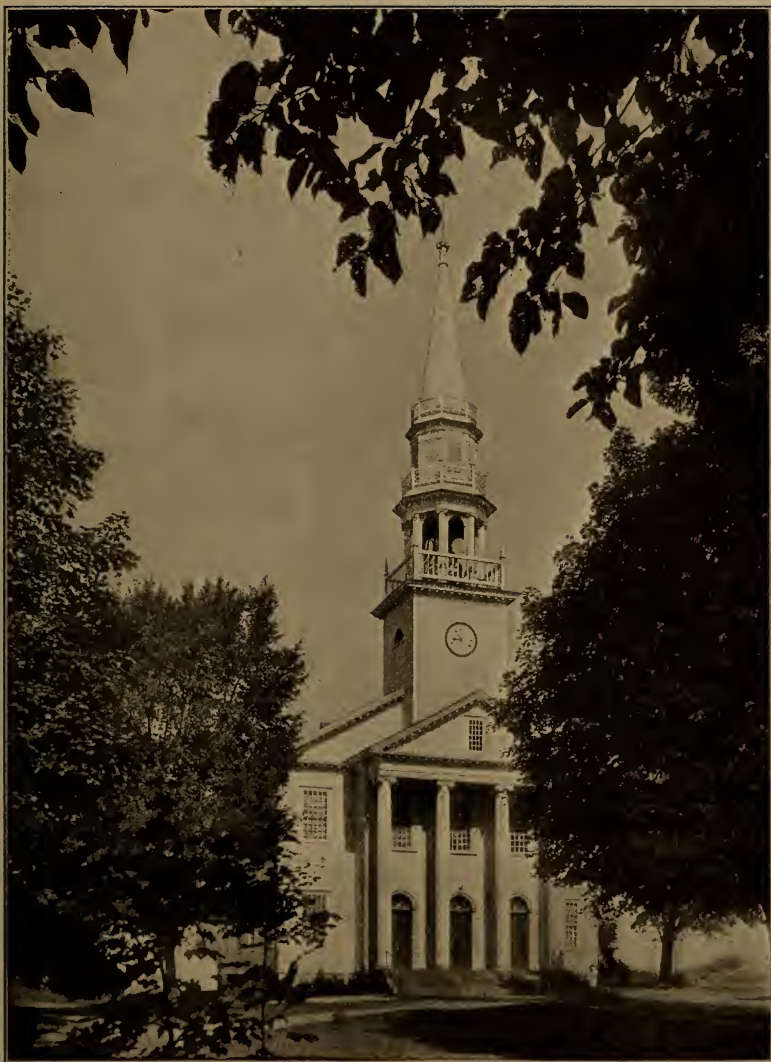
Hall & Winton, Builders, 1826.
